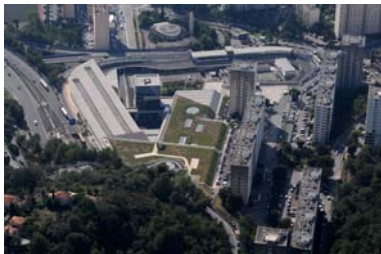
Multimodal Center – Nice Tramway
