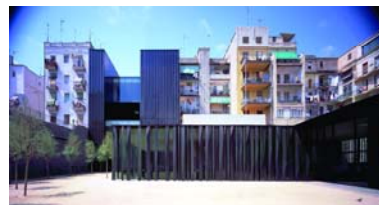
Library, Senior Citizens' Centre and City Block Core Zone, Sant Antoni's District
